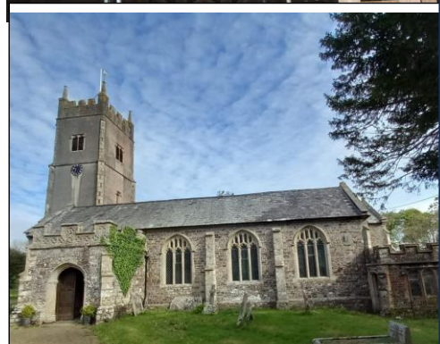
← Churchwarden's photo of Chawleigh church after roof/guttering repairs and scaffolding taken down.
