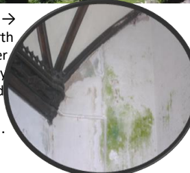
→ Damp, north west corner before gully repairs and interior decoration.
