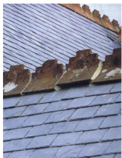
Bat slates in ridge
